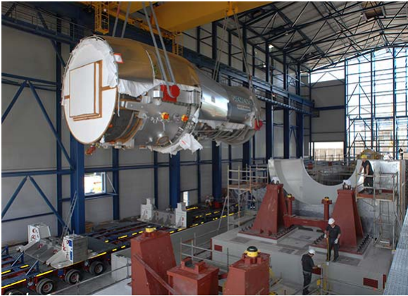
340 MW Siemens Gas Turbine
